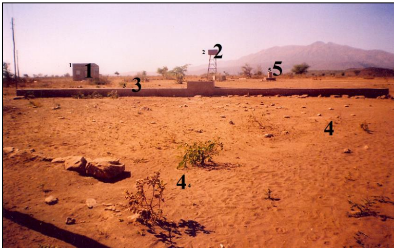
NB: 1=Destroyed water pumping generator; 2=unfunctional water tanker at hill of water tower; 3=cattle trough for water consumption; 4=degraded land around the borehole and 5=unfunctional water point.
