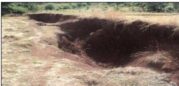
Fig 10. Eroded Land in Sigeda Kebele in Soro Woreda, Hadiya Zone, SNNPR
